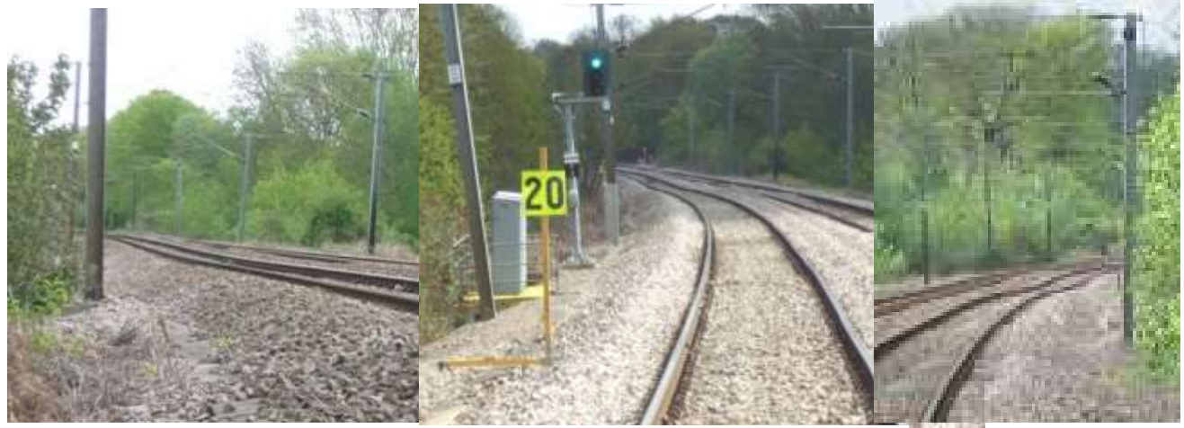
Long Dip in track – Alignment Fault
